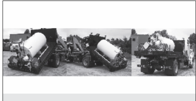
Figure 2.2 Hoisting Slide-in Unit for Installation in truck bed
